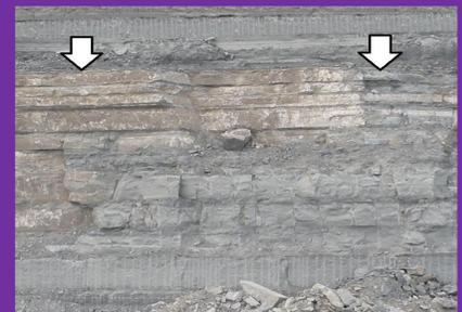
Fig. 4. A front view of the bench face. The arrows refer to the survey grid limits, 8m far from the face.
